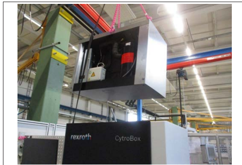
Fig. 14: Lifting the compressor cooler
